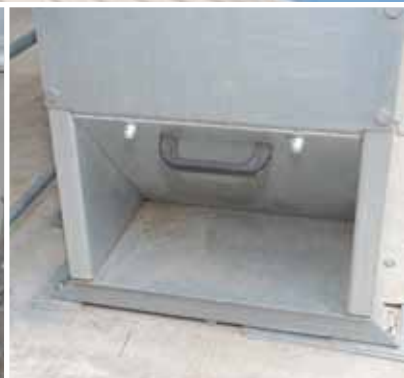
Access to elevator boot emptying.
