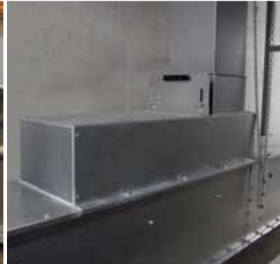
Intermediate Inlet with capacity control.
