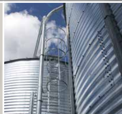
Pipe assembly for filling outdoor steel silos.
